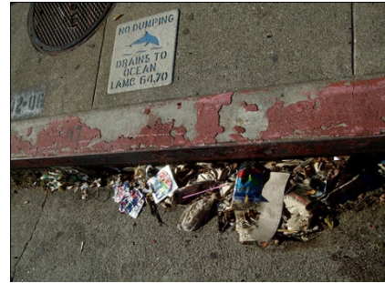
Figure 4 - Litter found in gutter
